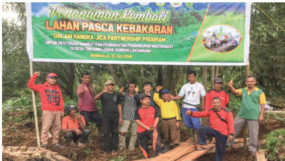
Weir construction in collaboration with residents
