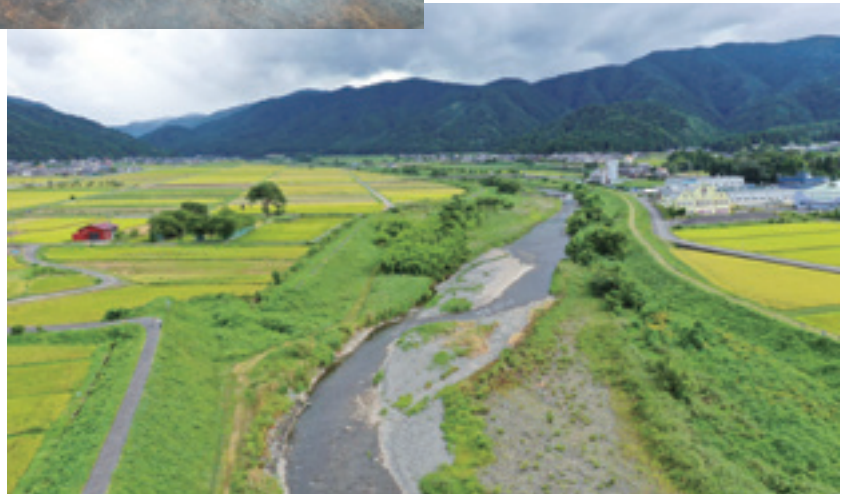
Photo 2 : Kasumi-tei (open levee), a traditional measure against riverine flood, remaining in the Kitagawa River (Fukui Prefecture). Many open levees still exist in this river and perform multiple functions including flood control and supporting biodiversity and ecosystem services in the watershed. Photo taken in September 2020.
